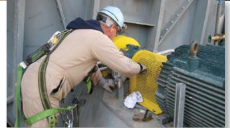
Coupling & Sheave Alignment
